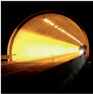
Before: 600W High Pressure Sodium 150W High Pressure Sodium
